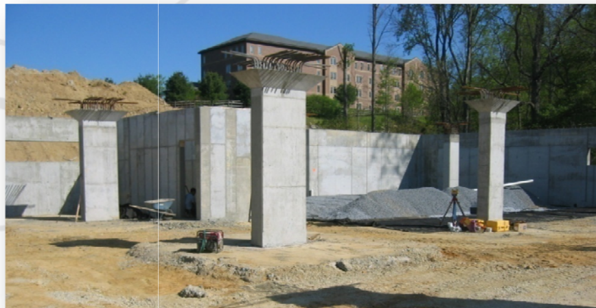
Figure 2: Wellington Condominium's Foundation
